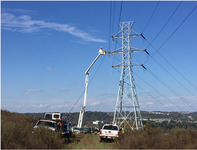
Figure 8: One side of a double circuit 138 kilovolt (kV) transmission line reconducted using 795 ACSS conductor and toughened glass insulators; courtesy of Duquesne Light Company.
