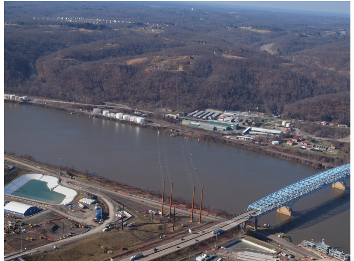
Figure 3: 3M ACCR conductor used to reduce sag and limit pole heights, which were the result of the long span lengths and difference in elevation; courtesy of Duquesne Light Company.
