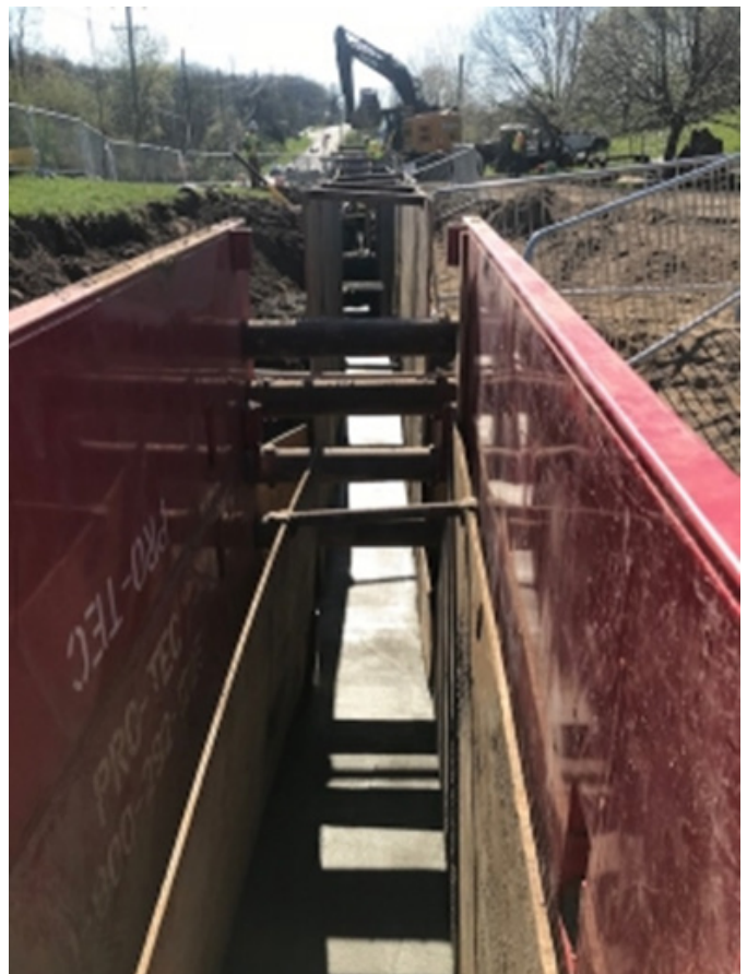
Figure 6: Underground duct bank construction; courtesy of ITC Holdings, Corp.
